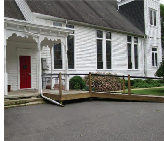
Two rain gardens can be installed to capture, treat, and infiltrate stormwater runoff from the roof. Downspout planter boxes can be constructed along the building to allow roof runoff to be reused. A preliminary soil assessment suggests that more soil testing would be required before determining the soil's suitability for green infrastructure.
