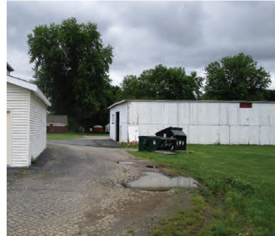
Porous pavement can be installed along the parking spots in the back lot of the building. The downspouts currently empty onto asphalt which is impervious and does not aid in infiltration. A preliminary soil assessment suggests that the soils have suitable drainage characteristics for green infrastructure.
