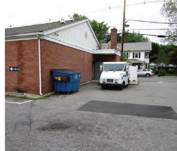
Porous pavement can be installed to collect stormwater from both the disconnected downspouts as well as from the parking lot surface. A preliminary soil assessment suggests that more soil testing would be required before determining the soil's suitability for green infrastructure.
